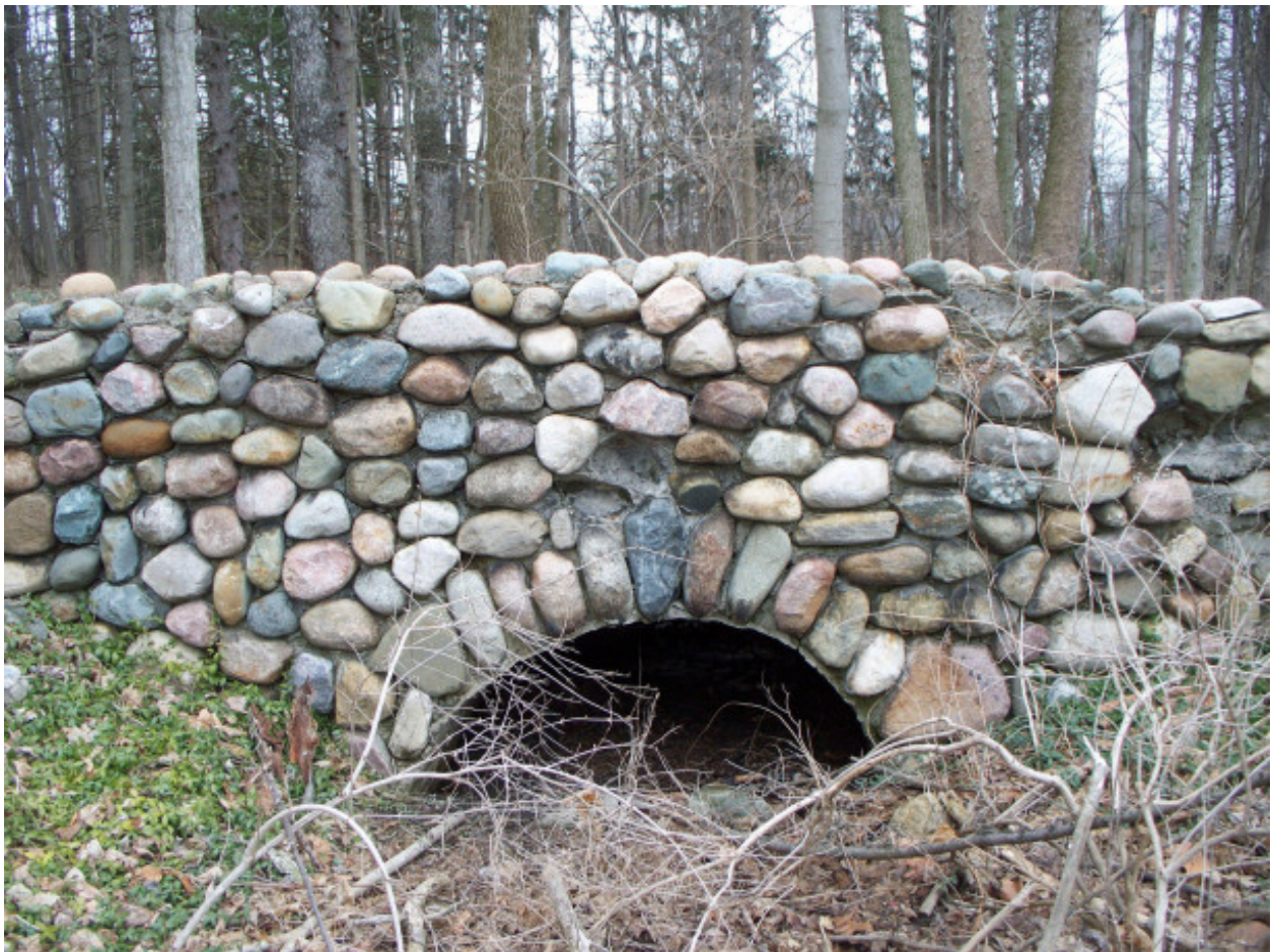
A fieldstone bridge over a gully on the property led to a single-family residence that once stood on this prominent corner (2013 photo by Sharon Butsch Freeland)
